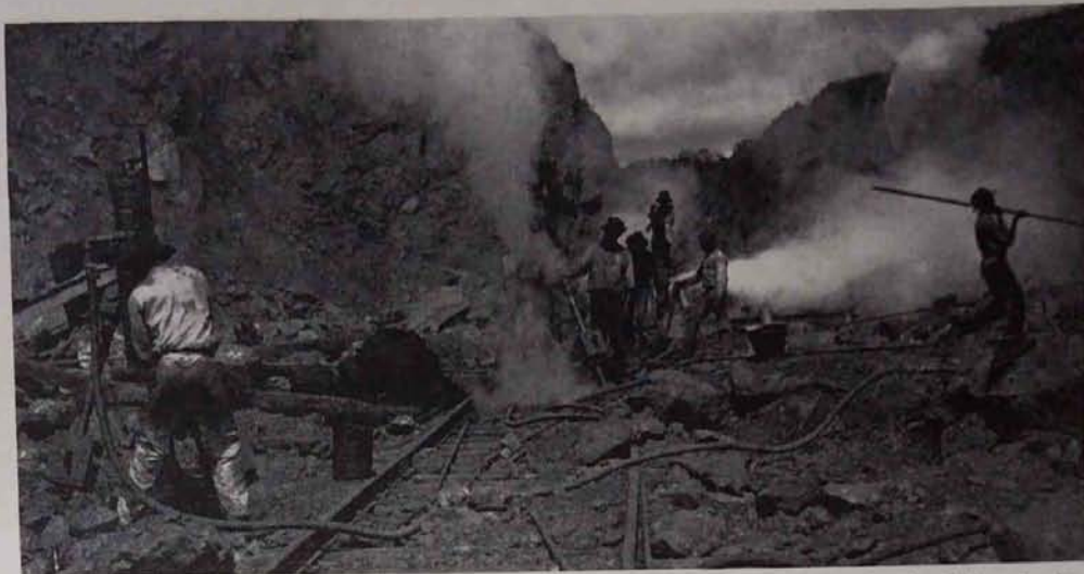
MAN OVER NATURE. Hacking away with steam drills and shovels, U.S. construction crews, like this one in the Bas Obispo Cut, moved more
